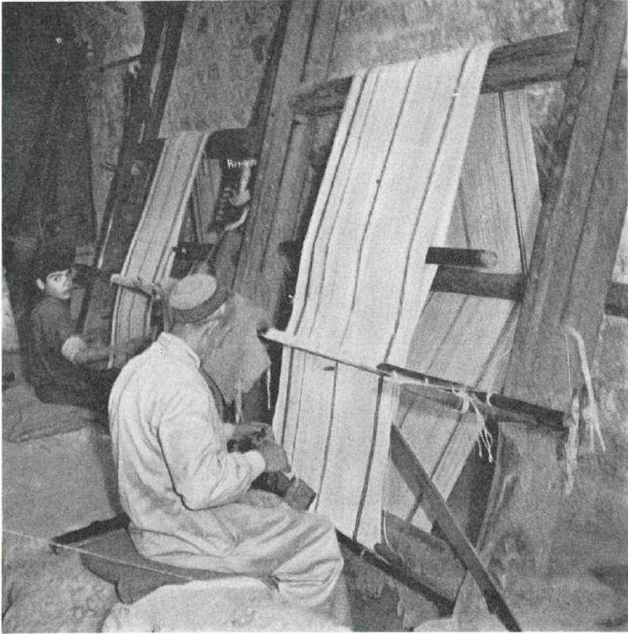
Fig. 38. Tubular loom with three beams put up with a short cotton warp for one sack. From an open workshop. The weaver sits on the floor with his legs placed in a pit. The photograph is taken from the street in Hama, 1961. (M. Hald fot.).
